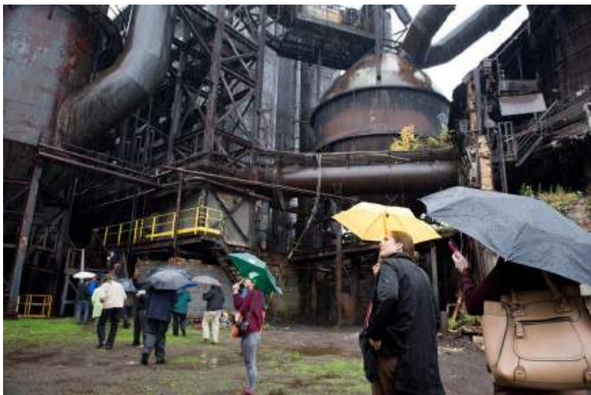
Relics of the Past: The Carrie Furnace is a former blast furnace located near Pittsburgh. At its peak, it produced 1000 to 1250 tons of iron per day, and it now serves as a historical site open for tours.
